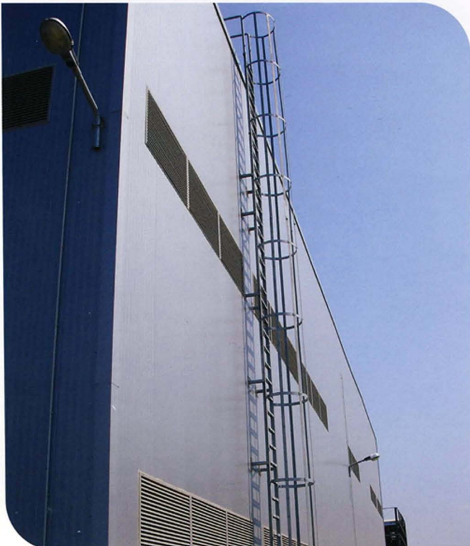
Ladders with or without safety cage, acc. to DIN 24532.
